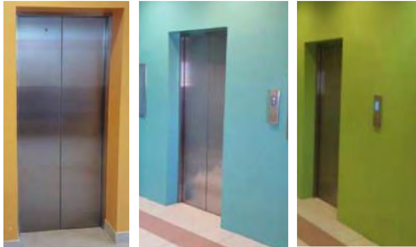
Naggo Head elevator installation
